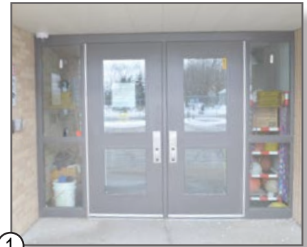
① HOLLOW METAL DOORS & HOLLOW METAL FRAME
