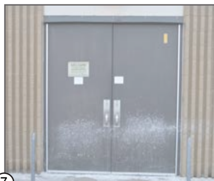
⑦ HOLLOW METAL DOORS & HOLLOW METAL FRAME
